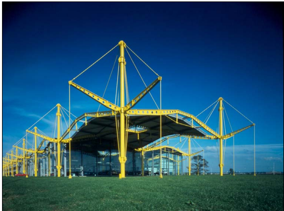
Figure 1.6 External structure supporting a single storey building
