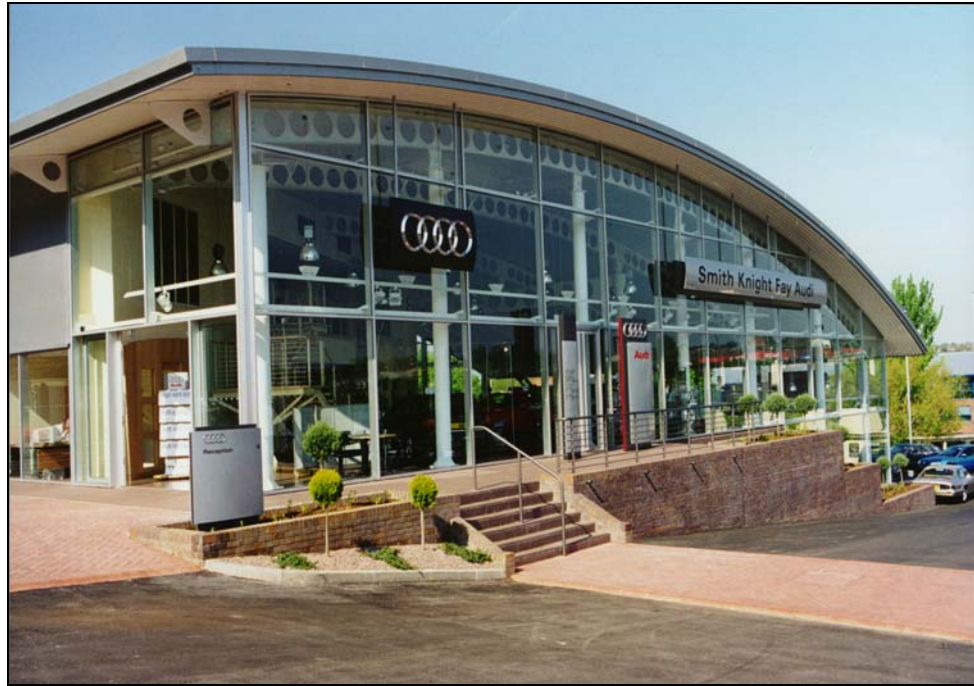
Figure 1.3 Use of curved cellular beams in a portal frame
