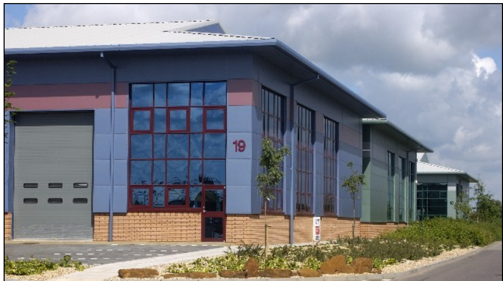
Figure 1.8 Large windows and use of composite panels with “dado” brick wall
