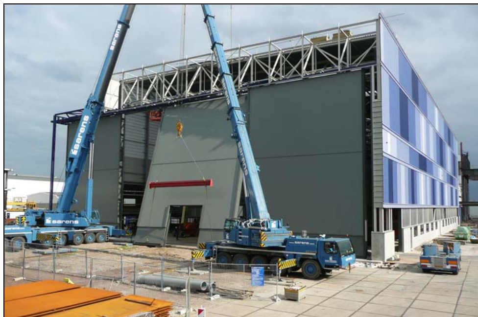
Figure 2.6 View of doors being lifted into place in Hollandia's building in Krimpen aan den IJssel
