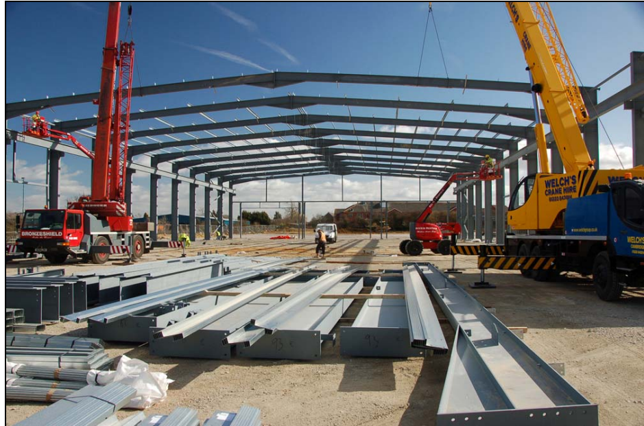
Figure 2.1 Portal frame during construction
