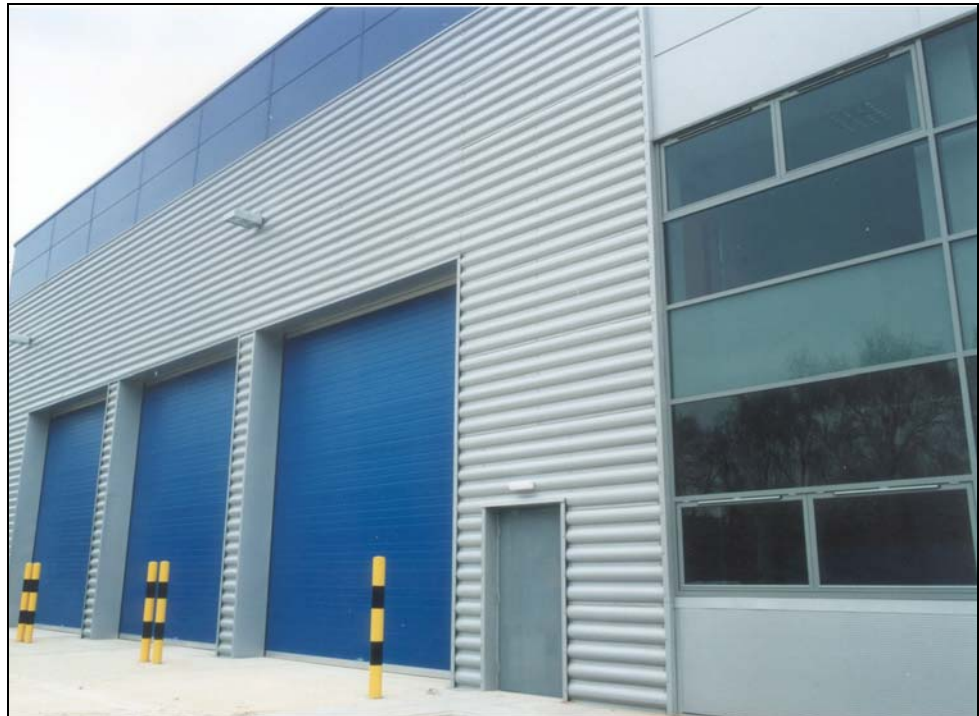
Figure 1.7 Horizontal spanning sheeting
