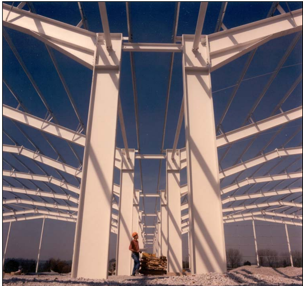
Figure 1.2 Multi bay portal frame structure
