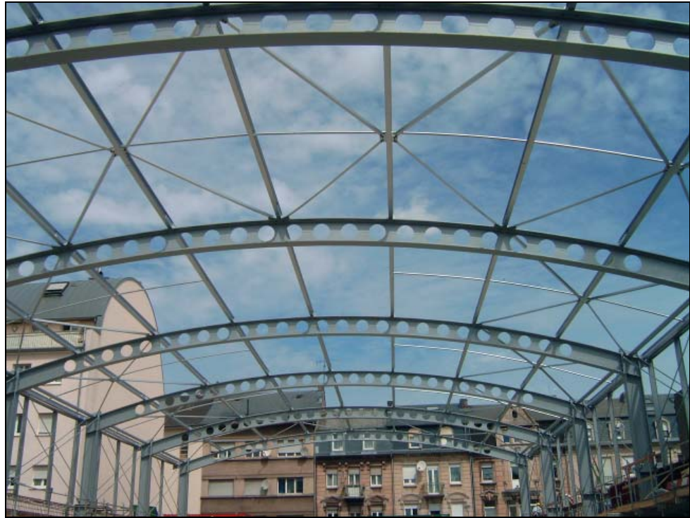
Figure 2.3 Portal frame structure using curved cellular beams
