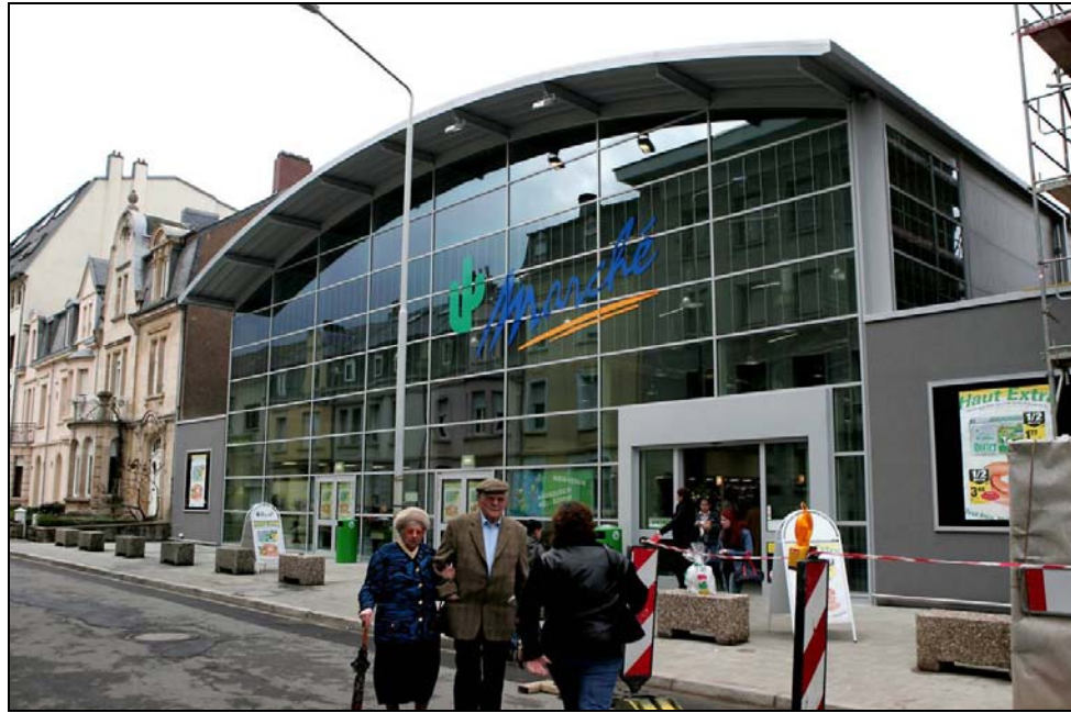
Figure 2.2 Supermarket in Esch , Luxembourg using curved cellular beams
