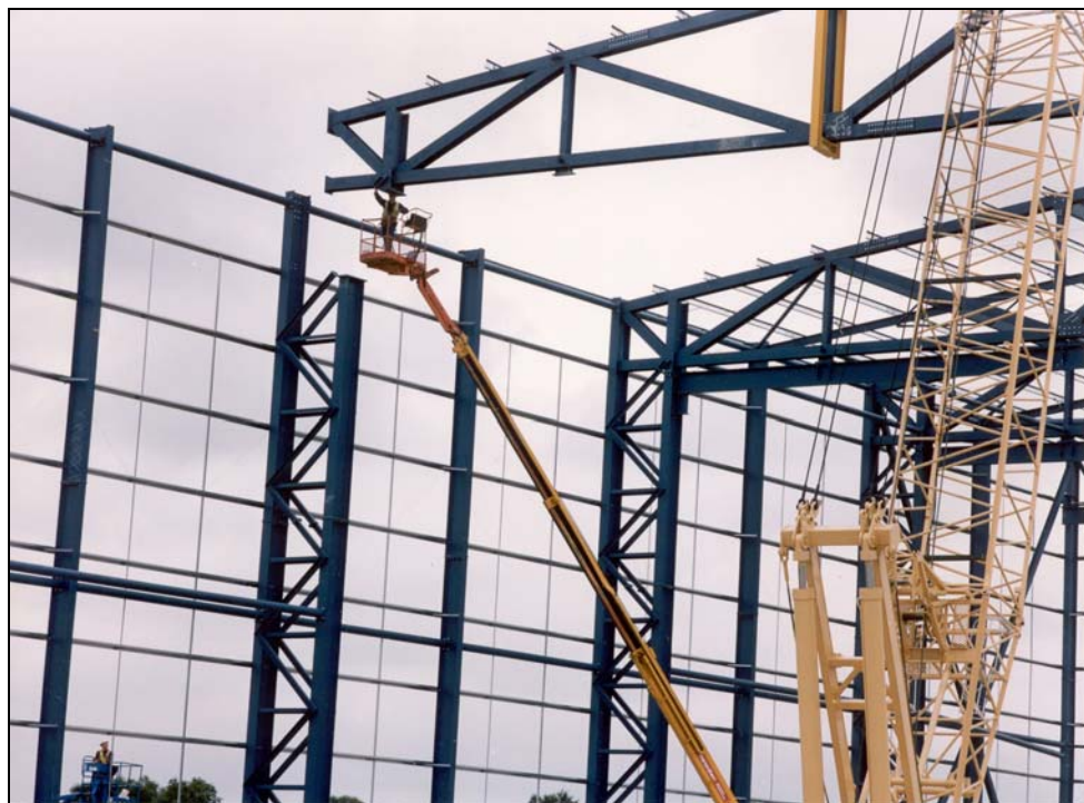
Figure 1.4 Roof trusses and built-up columns
