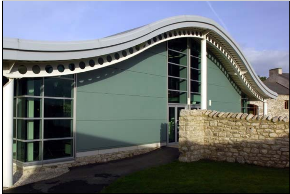
Figure 1.5 Curved cellular beams used in a leisure centre
