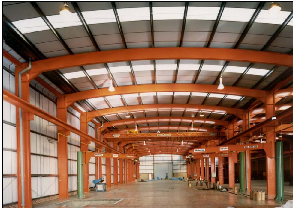
Figure 3.22 Curved beams used in a portal frame
