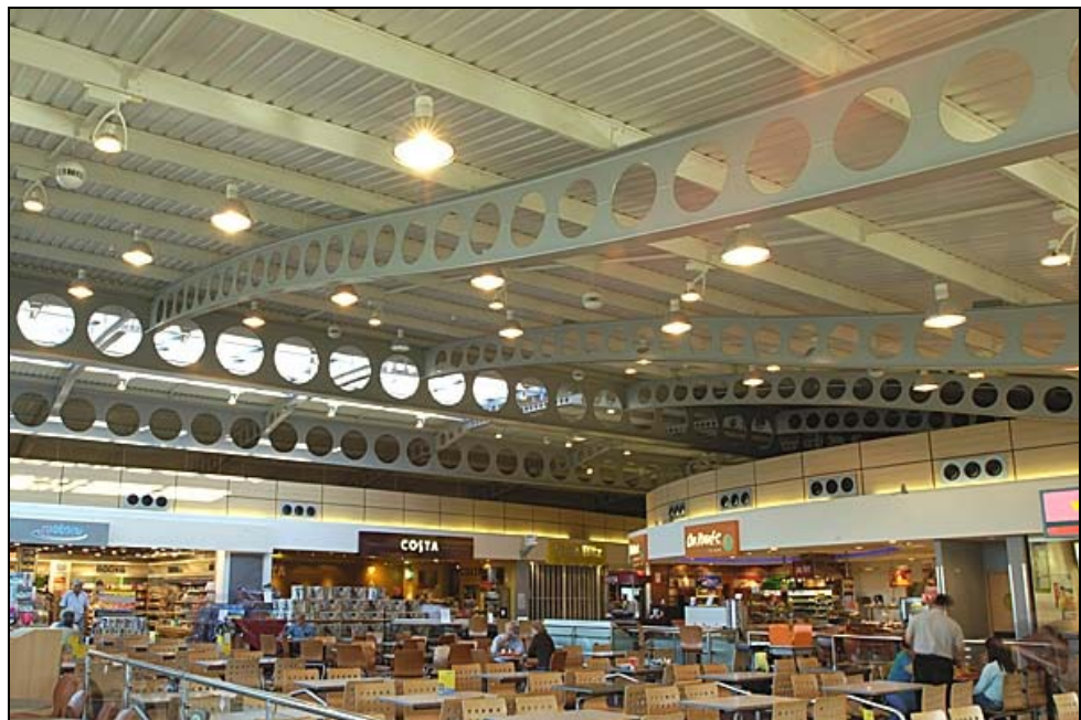
Figure 2.4 Double curved cellular beams and primary beams
